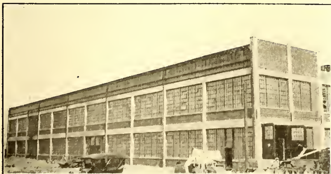
DETROIT UNITED WOOD SHOP—WEST SIDE OF BUILDING
